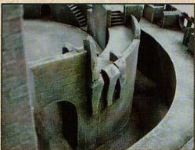
Inside the walls.
